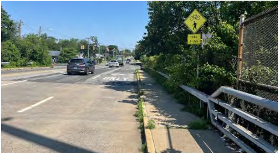
Figure 2. Connetquot Ave facing north.
