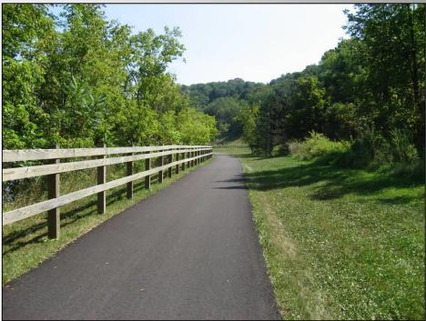
Standard trail is 10 feet wide with stone dust or asphalt surface
