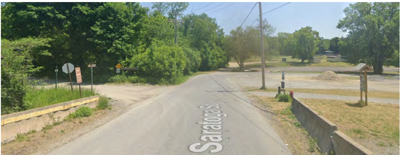
Lack of crossing infrastructure across Saratoga St/Red's Rd
