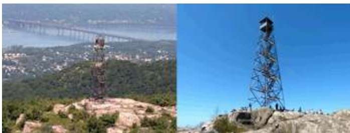
The fire tower before (left) and after (right) restoration. Photos by David Rocco.
