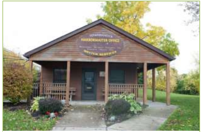
Harbormaster Office in Tonawanda, offering services to boaters and possibly cyclists in the future
