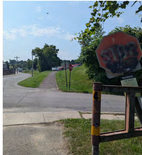
Broad St trail crossing featuring vandalized sign and lack of crosswalk.
