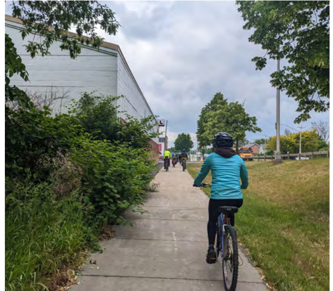
The Mohawk River Trail does not provide a standardized "multi-use trail" experience and is subject to overgrown vegetation.
