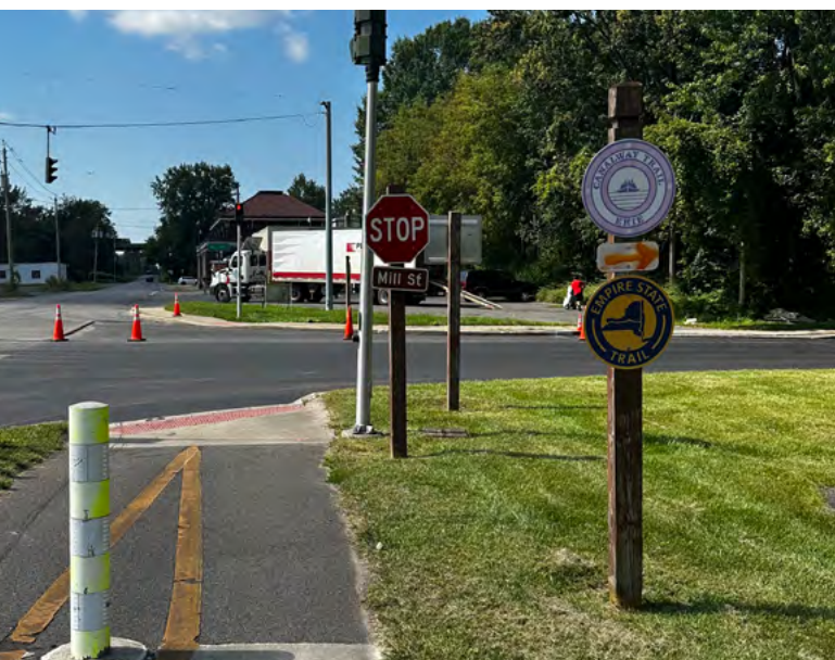
Faded and damaged signage where the trail turns onto Mill Street. Photo credit David Hinman.
